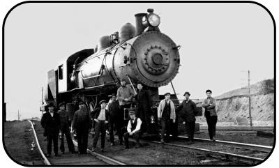
This train crew is working the "Hump Engine". Notice that that track to the left rear goes up as it disappears in the distance. The engine crew consisted of two men. There would also be a conductor and a switchman. The rest of the crew would be brake men who would ride the cars down the track and apply brakes as needed. (year unknown)
